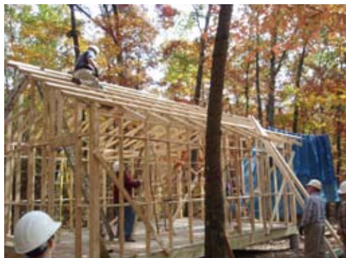
Raising the new cabin at Opequon
